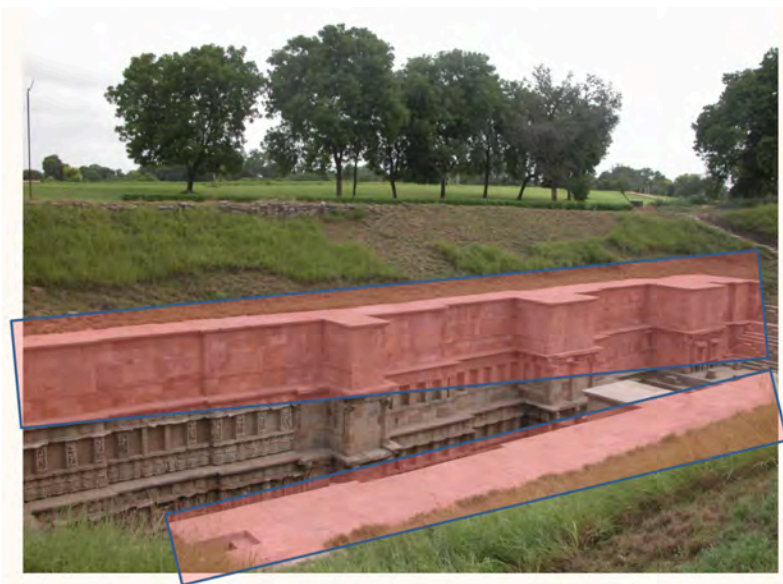
Figure 29 - Added retaining walls (ASI, p.127)
